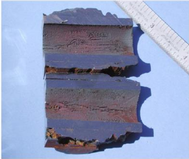
Boiler tube corrosion
